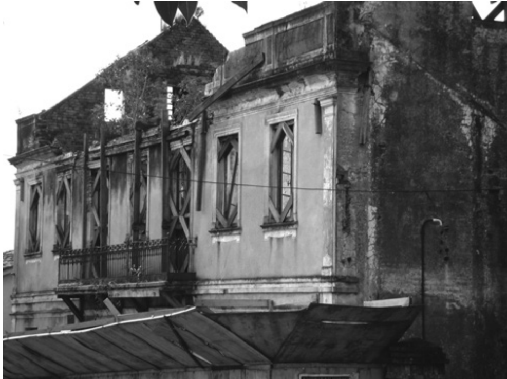
Figure 1. Home for Girls, facade before the restoration. Image by the author.
