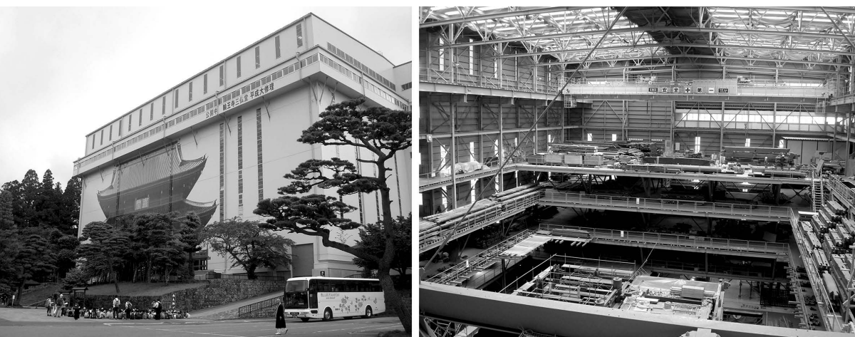
FIGURE 3. THE RINNŌJI TEMPLE, NIKKO, TOTALLY DISMANTLED FOR ITS RESTORATION, 2014.
