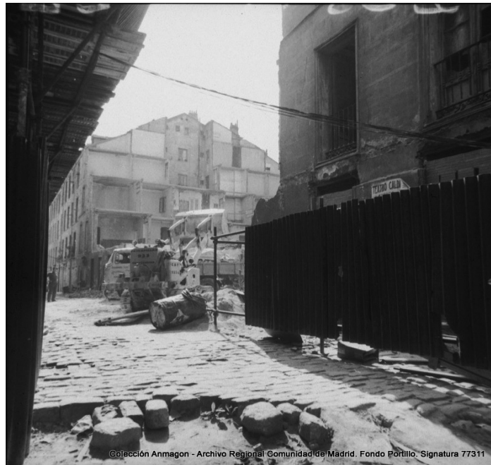
FIGURE 3B. VIEW OF CALLE DE HERMOSA IN THE NEIGHBORHOOD OF LAS POZAS, MADRID, DURING THE PROCESS OF DEMOLITION OF THE HOUSES, OCTOBER 1969. Image: Collection Anmagón, Archivo Regional de la Comunidad de Madrid, Fondo Portillo, signatura 77311-023.
